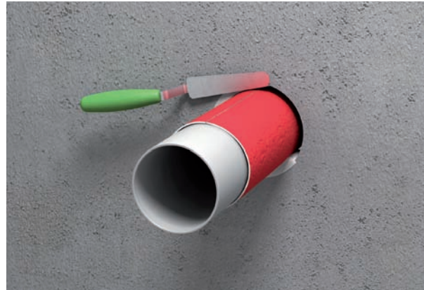
Close remaining or ring gap in a flue gas-tight manner
