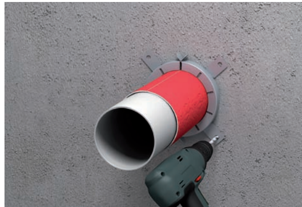
If necessary, mark and set up the fixing points
