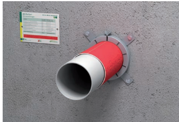
Fill in the identification plate as supplied and attach next to the fire-retarding seal.
